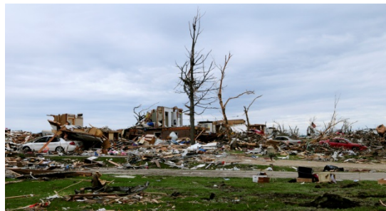
Figure 11. Debris on Private Property
