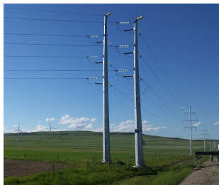
Replacing power poles with higher-rated poles prevents future damage.
